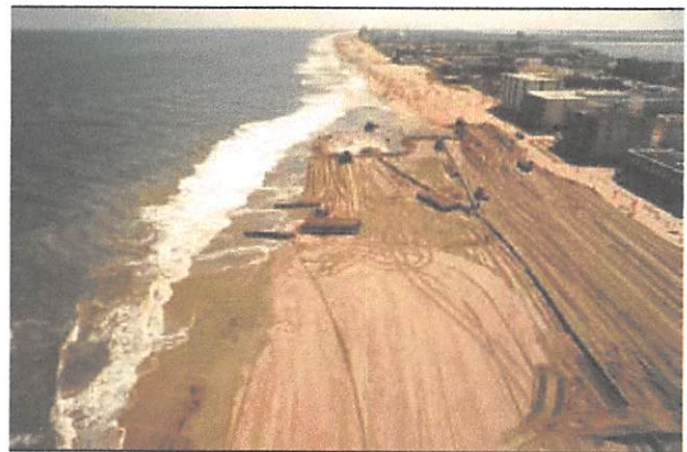
Beach nourishment projects repair erosion while increasing the distance between vulnerable coastal infrastructure and breaking waves, while dunes protect against wave energy and flooding. Source: http://marine.rutgers.edu/geomorph/oceanicityfill.jpg
